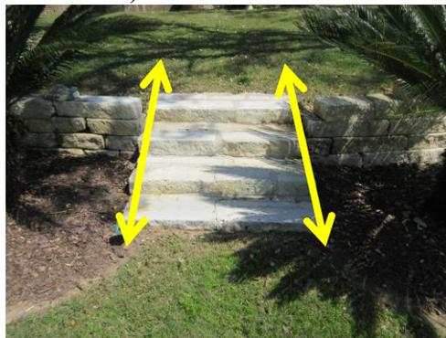
Per current accepted trade practices, a hand rail should be added to the exterior steps. Hand rails should be provided when an elevation change of 4 or more risers occur.
