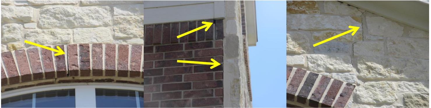
Cracks were observed in the exterior brick/stone walls of the structure. This implies that some structural movement of the structure has occurred, as is typical of most structures.
