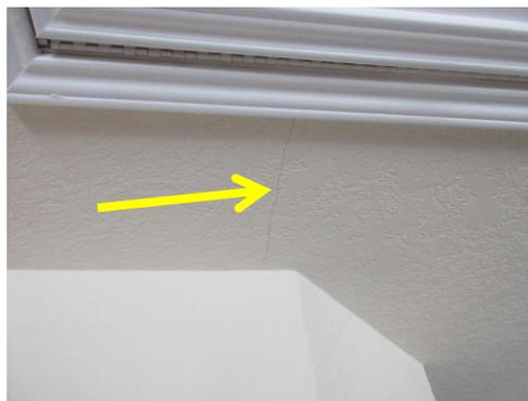
Crack(s) were observed in the ceiling of the structure. This implies that some structural movement of the building has occurred, as is typical of most structures. (See photo above)
