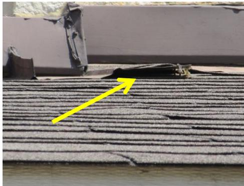
Lack of maintenance and sealing of all flashing material may be expected to contribute to roof leakage points. Buyer may want to consider additional roof inspections based on the age, unknowns, and or levels of assumed risk.
