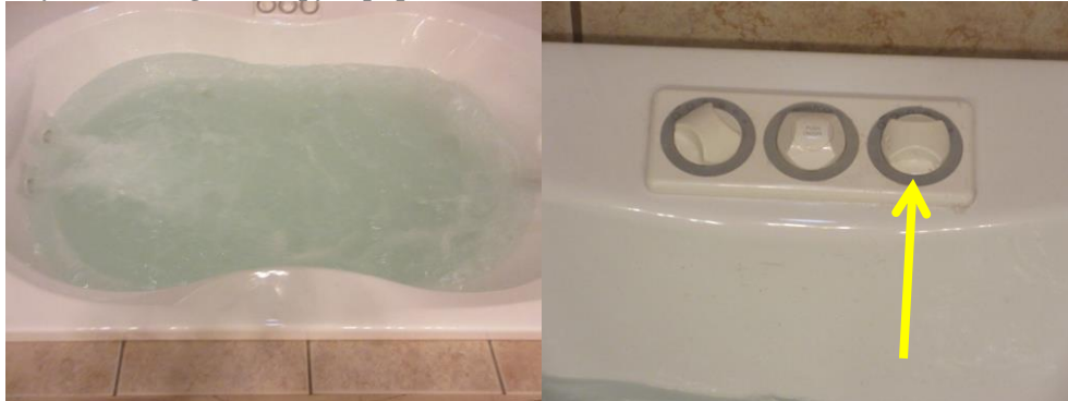
A damaged control knob.
