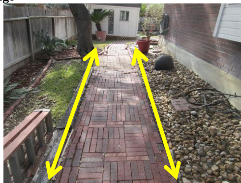
Trip hazards noted all around the structure.
